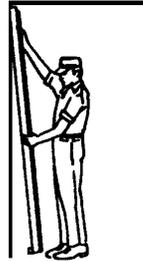
2. Drive sill anchors on to bottom of both jambs.
