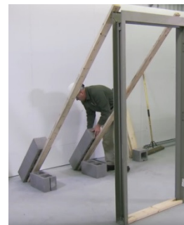
Figure 8 – Temporarily brace frame
