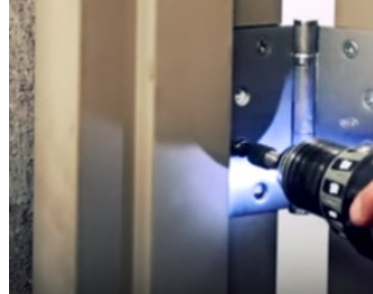
Figure 20 – Install Ives hinge first in top location
