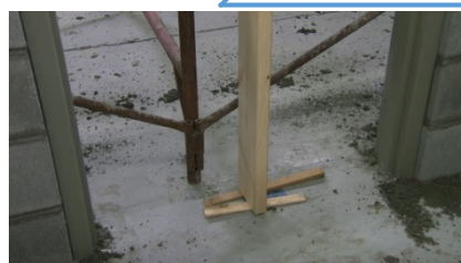
Figure 13 – Support head with a vertical brace on any head over 42” long. Shim as needed to keep head level
