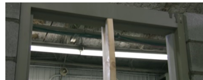
Figure 12 – Check for plumb, level and square every time you make an adjustment
