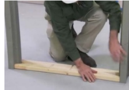
Figure 6– Spreader placed betw Strike Jamb & Hinge jamb
