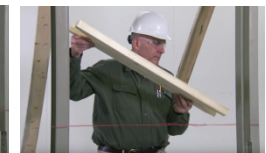
Figure 9a – Add mid height spreader bar
