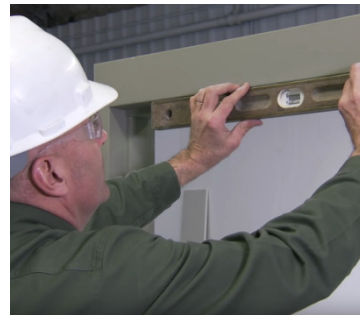
Figure 12 – Check for plumb, level and square every time you make an adjustment
