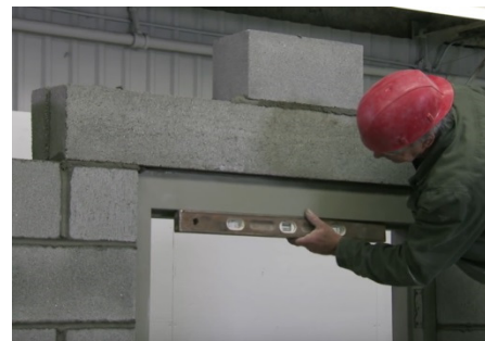
Figure 15 – Typically a high PSI concrete lintel is used. Check that plumb, level and square is maintained to ensure no sagging
