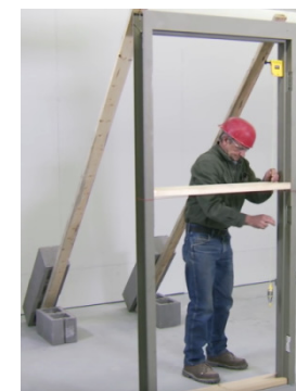
Figure 10 – Mason should check plumb, level, square before beginning
