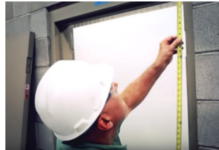
Figure 17 – Verify hinge locations
