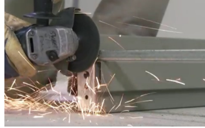
Figure 5– Properly grind off shipping bar
